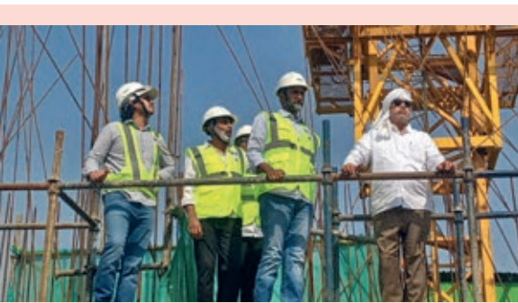
ASN Raju, Wholetime Director and Harsha Varma, Director (Projects) visited WWTF Project Malad on 16 December 2025
